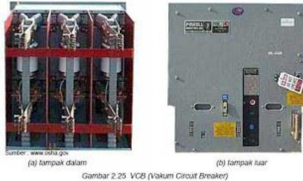
Gambar 2.25 VCB (Vacuum Circuit Breaker)
