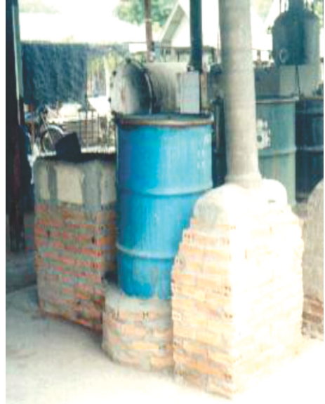
Fueled by wood shavings
