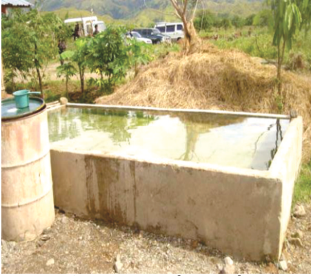
A concrete soaking tank
